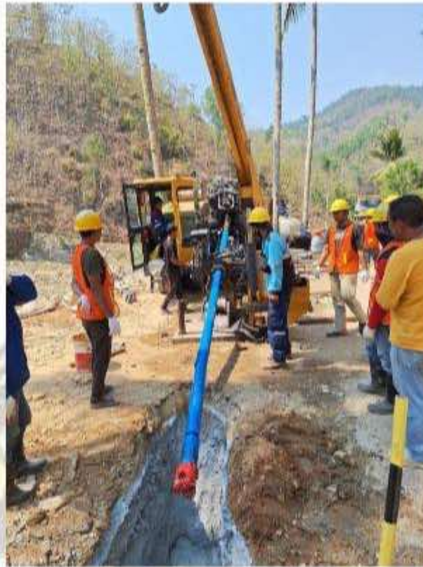
Gambar 2.6 Metode Pekerjaan Horizontal Directional Drilling
