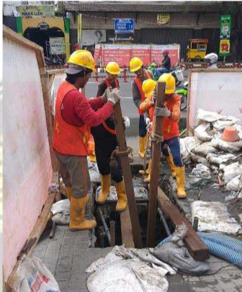
Gambar 4.3 Metode Boring Horizontal Manual (Sumber : PT PGAS Solution)
