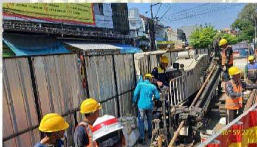
Gambar 4.4 Metode Horizontal Directional Drilling (Sumber : PT PGAS Solution)
