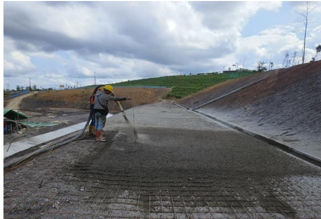
Gambar 2.16 Metode Wet Shotcrete
