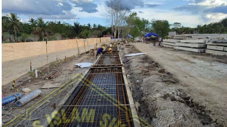
Gambar 4.10 Proses Penulangan Concrete Panel
