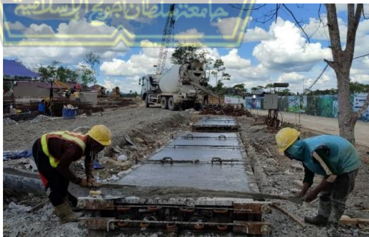
Gambar 4.11 Proses Pengecoran Panel
