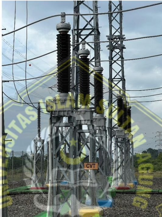
Gambar 2. 5 Trafo Tegangan (Potential Transformer)
