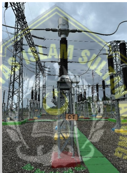
Gambar 2. 6 Trafo Arus (Current Transformer)
