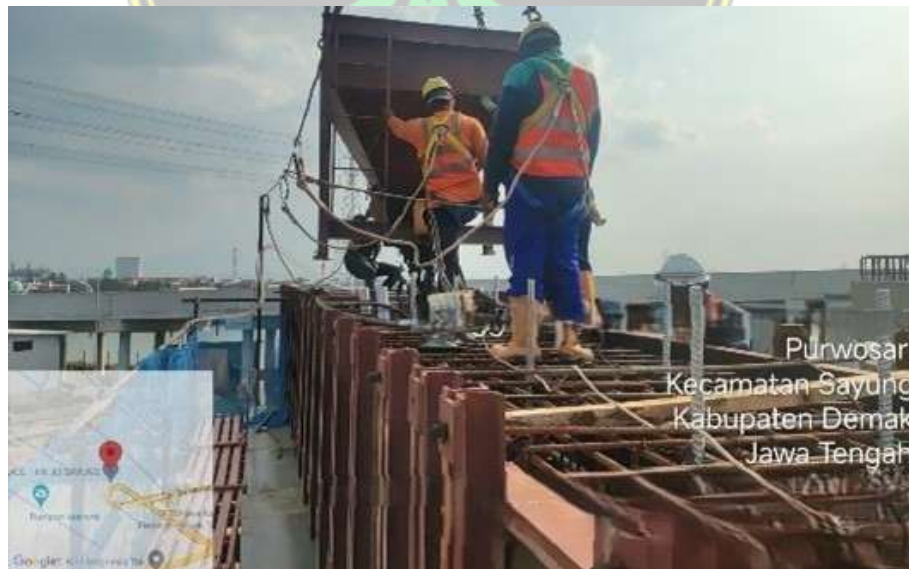
Gambar 4.44. Pengecoran Mass Concrete Pile Head
