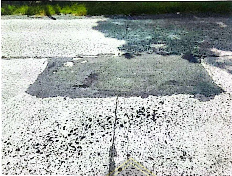
Gambar 4.9. Tambalan ( Patching end Utiliti Cut Patching )
