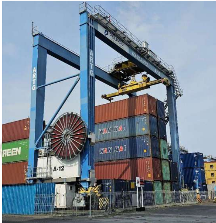
Gambar 2. 6 Automated Rubber Tyred Gantry Sumber : Dokumen Pribadi, 2024
