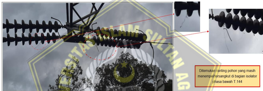
Gambar 4.36 Eviden lapangan gangguan PHT Ombilin-Indarung
