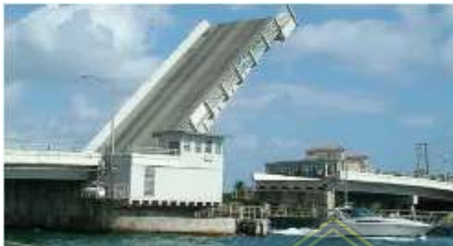
Gambar 4.5 Single Leaf Bascula Two River Bridge Wisconsin
