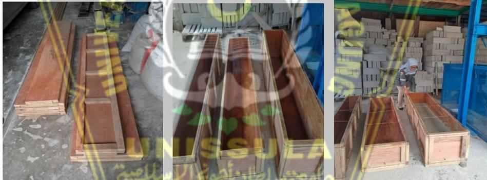
**Gambar 4.26:** Bekisting Mortar Busa
