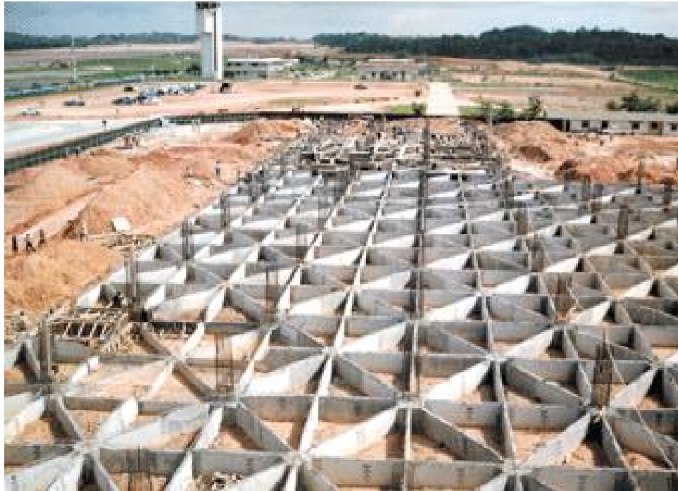
Figure 1.4. Preparing Sarang Laba-Laba foundation use as subgrade of the pavement
