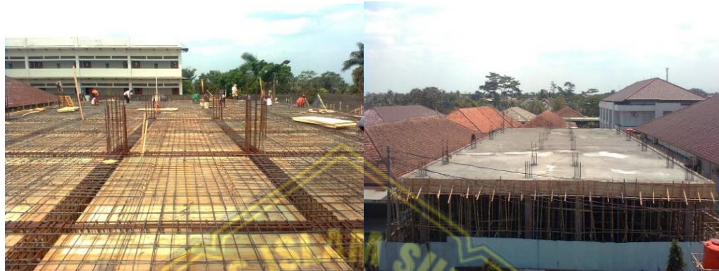
Gambar 4.16 Pelat Cast in place
