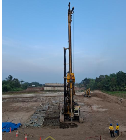
Gambar 4.3 Alat drilling rig pengeboran DCM PT Keller Ground Indonesia
