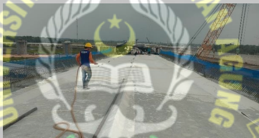
Gambar 4. 6 Proses Curing Beton
