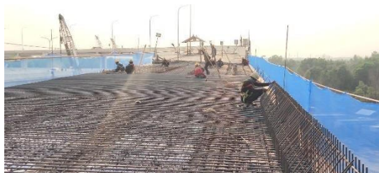
Gambar 4. 7 Proses Pembesian Parapet
