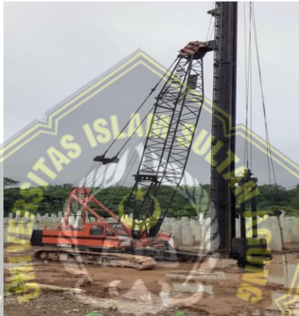
Gambar 2.7 Hydraulic Pile Driver
