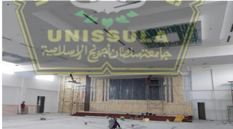
**Gambar 4.6** Instal Panel Videotron
