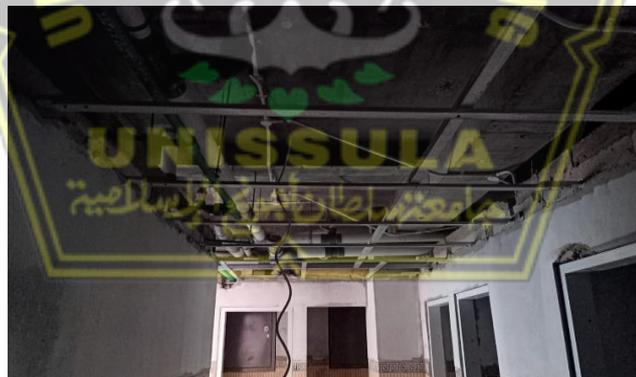
**Gambar 4.18** Rangka Hollow Alumunium
