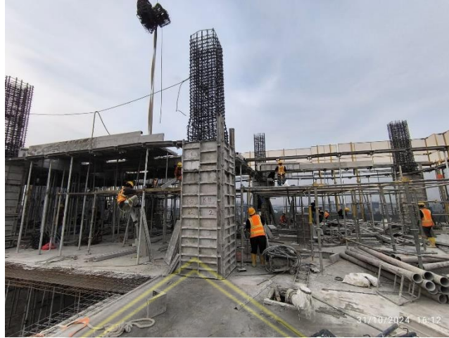
Gambar 2.3 Bekisting Aluminium
