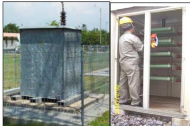
Gambar 2. 9 Neutral Grounding Resistor (NGR) [9]
