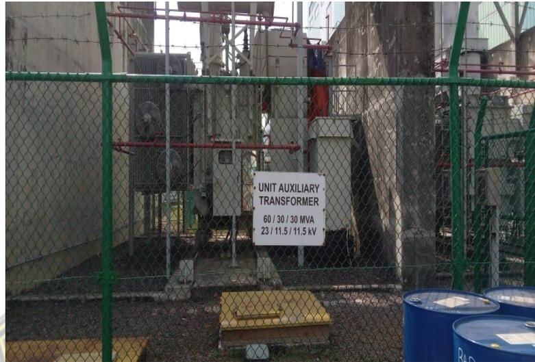
**Gambar 2. 2 Unit Auxiliary Transformer 30 MVA.**
