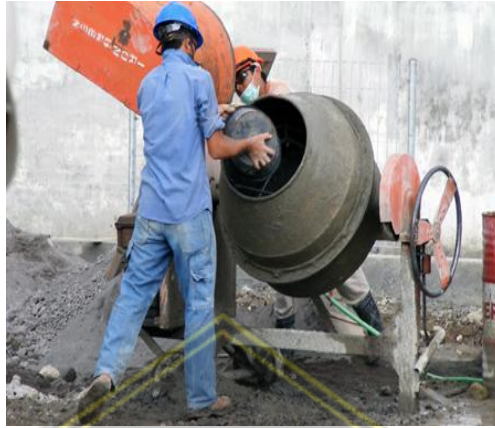
Gambar 3.7. concrete mixer Sumber: Google.com
