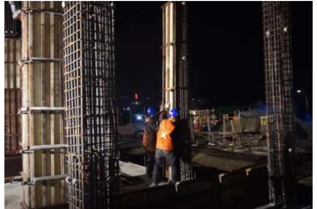
Gambar 3. 2 Bekisting Semi Sistem
