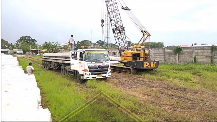
**Gambar 2.2.** Pengadaan *Corrugated Concrete Sheet Pile*
