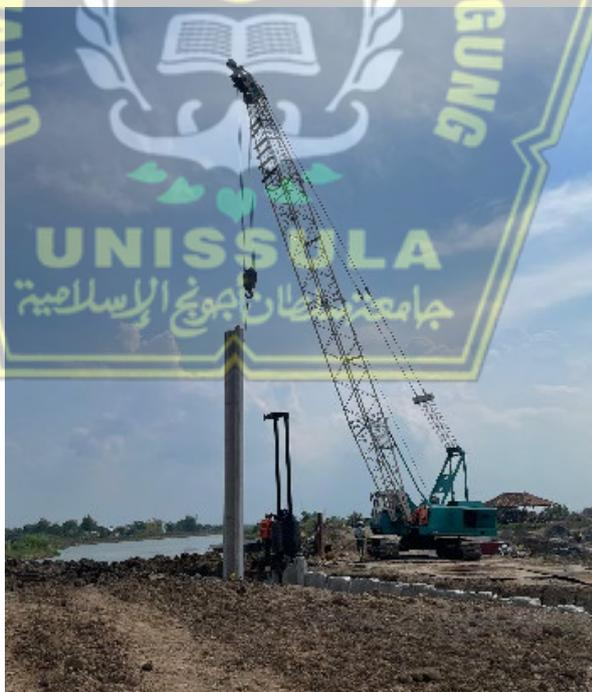
**Gambar 2.2.** Pengadaan *Corrugated Concrete Sheet Pile*
