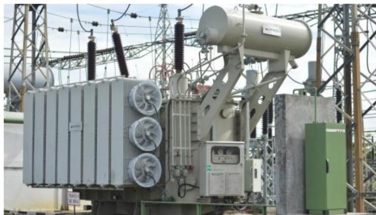
Gambar 2. 2 Transformator Daya [8]
