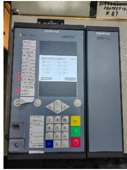
Gambar 3.4 Relai Siemens Siprotec 7SL87
