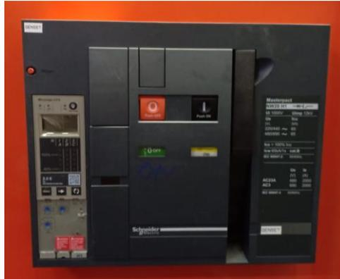
Gambar 2. 3. ACB (Air Circuit Breaker)
