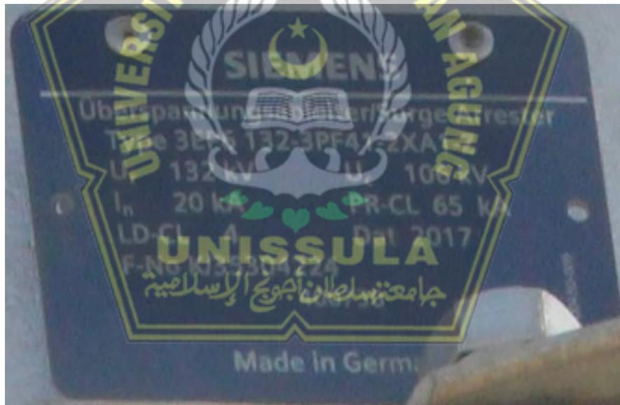
Gambar 3. 6 Nameplate lightning arrester gardu induk 150 KV New Batang
