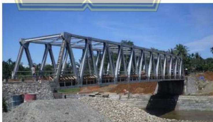
Gambar 2.16 Jembatan Warren Truss
