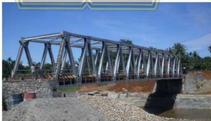
Gambar 2.16 Jembatan Warren Truss
