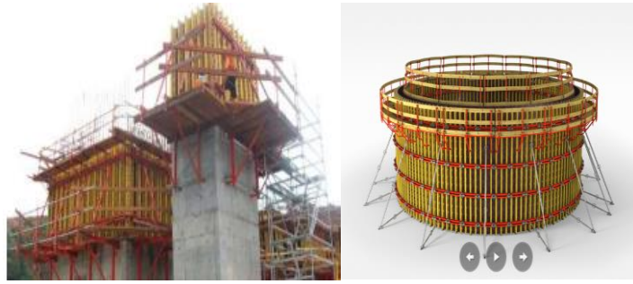
Gambar 2. 12 Pelaksanaan Sistem Peri Vario Column and Wall
