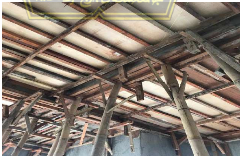
Gambar 4.17. Bekisting Plat Lantai Elv. +4.10
