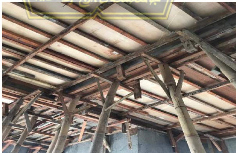
Gambar 4.17. Bekisting Plat Lantai Elv. +4.10
