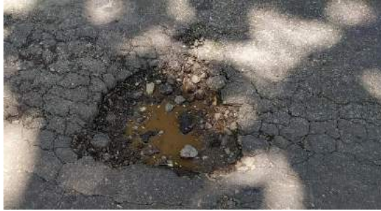
Gambar 2. 15 Lubang ( Potholes )
