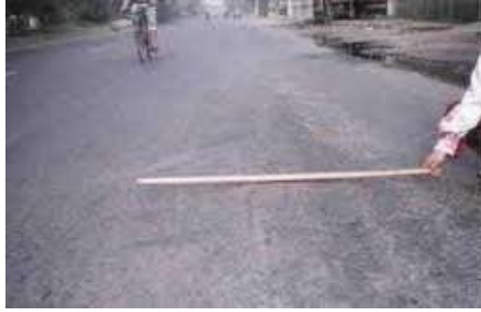
Gambar 2. 14 Jembul ( Upheaval )
