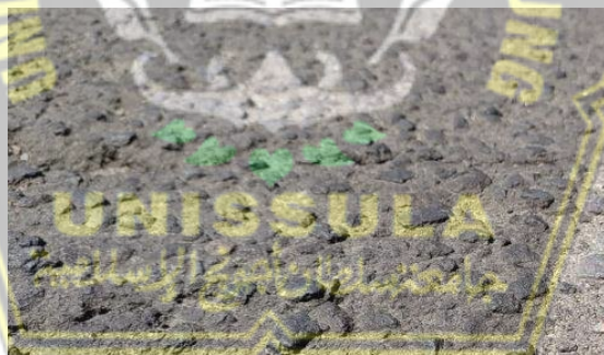
Gambar 2. 18 Pengausan ( Polished Agregat )
