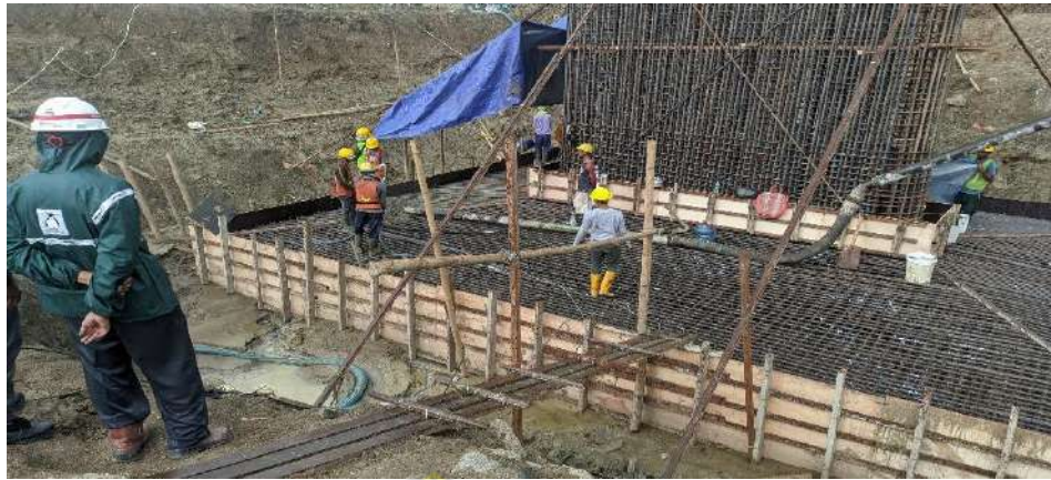
Gambar 2.20 Bekisting Konvensional
