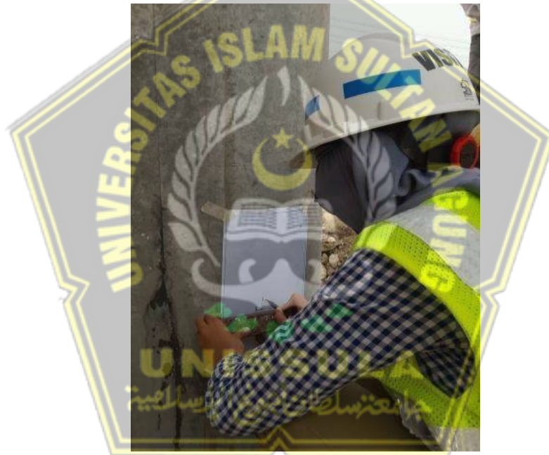
Gambar 2.17 Proses Kalendering Spun Pile.
