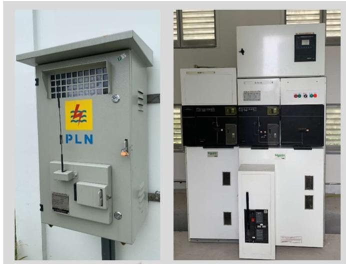
Gambar 4.33 KWH meter Pad panel induk PLN
