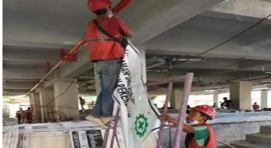
**Gambar 4.4** Memasang rambu-rambu keselamatan dan safety line.
