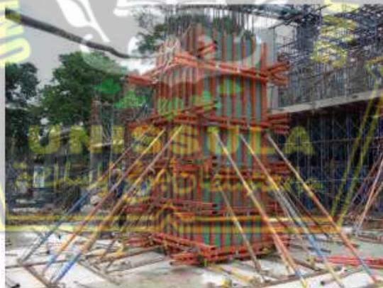
**Gambar 2.16** Bekisting Semi Sistem
