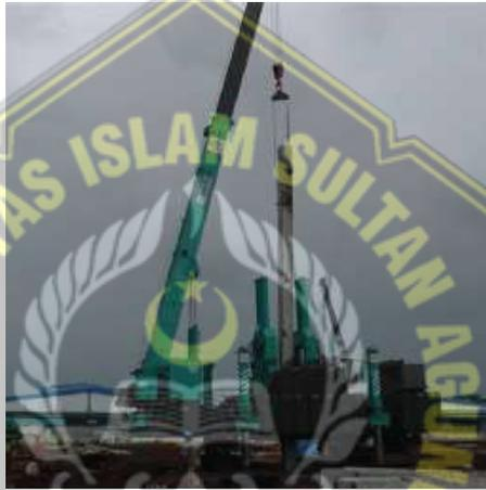
**Gambar 2.14** Mesin *Press in Pile*
