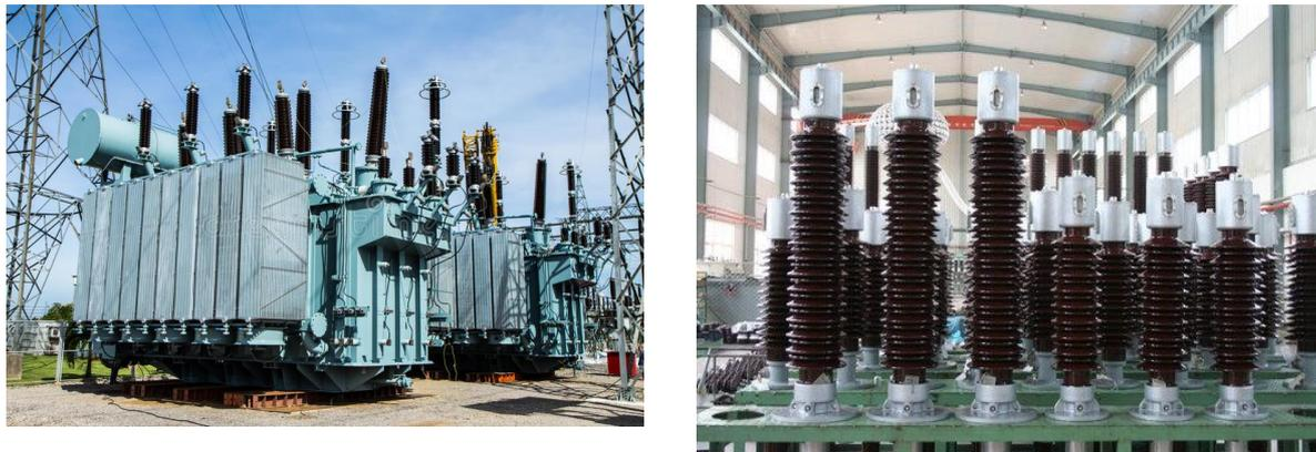
**Gambar 2. 9** Gambar Bushing Transformator
