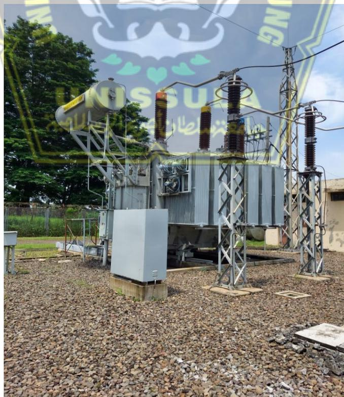
**Gambar 2. 5** Gambar Fisik Transformator 40 MVA
