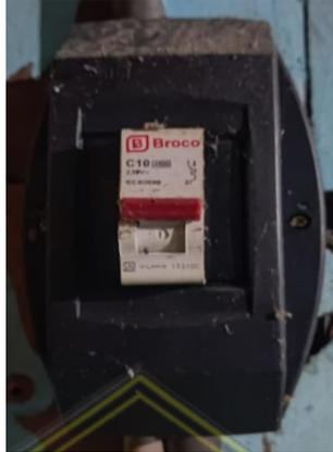
**Gambar 2. 11** Miniature Circuit Breaker (MCB)
