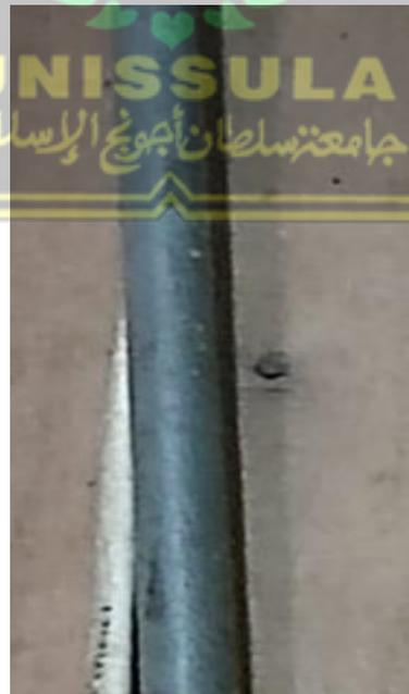
**Gambar 2. 9** Kabel Penghantar Instalasi Listrik Tipe NYA berlapis Pipa PVC
