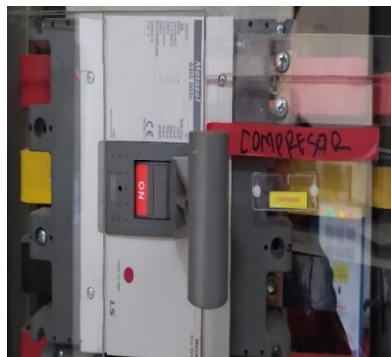
Gambar 2.4. Moulded Case Circuit Breaker (MCCB)
