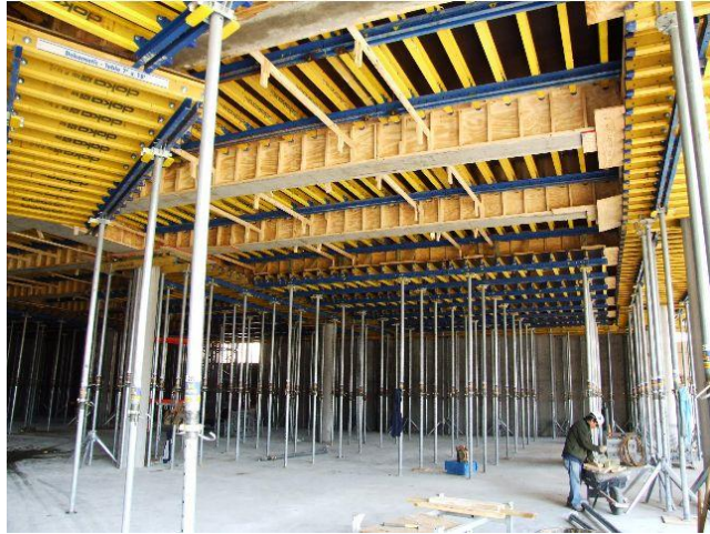
Gambar 2.16 Bekisting Semi Sistem. ( Sumber : https://binamarga.pu.go.id/ )
