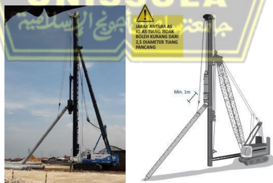
Gambar 2.7 Proses Penegakan Spun Pile.
