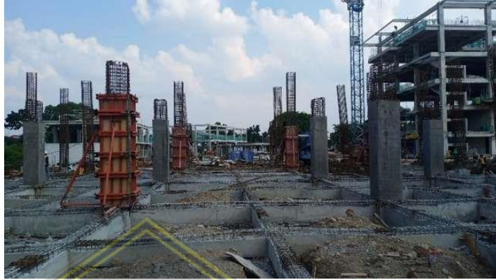
Gambar 2.7 Bekisting Kolom
