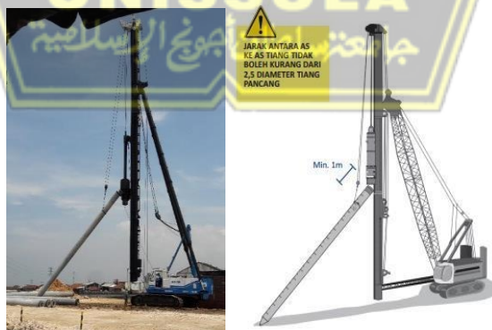
Gambar 2.7 Proses Penegakan Spun Pile.
