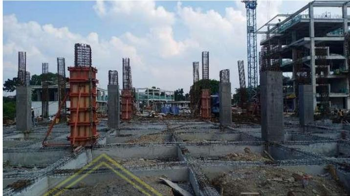
**Gambar 2.7** Bekisting Kolom
