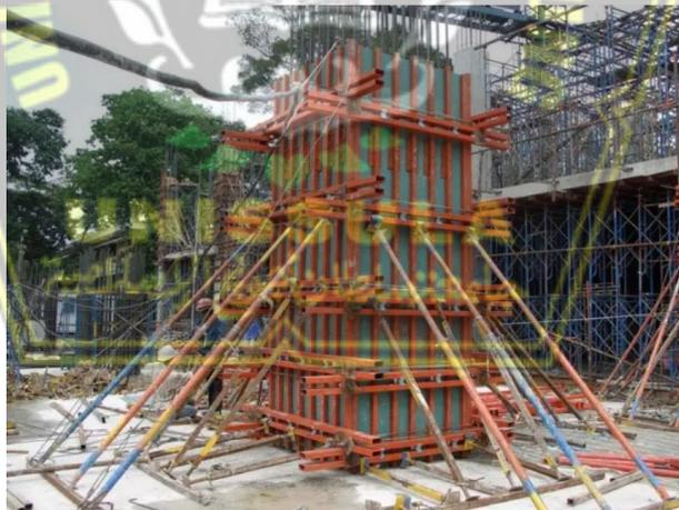
**Gambar 2.2** Bekisting Semi Sistem
