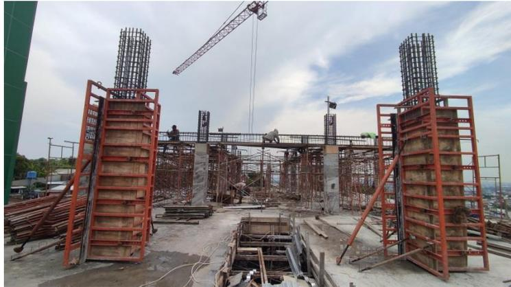
**Gambar 2.4** Bekisting Kolom
