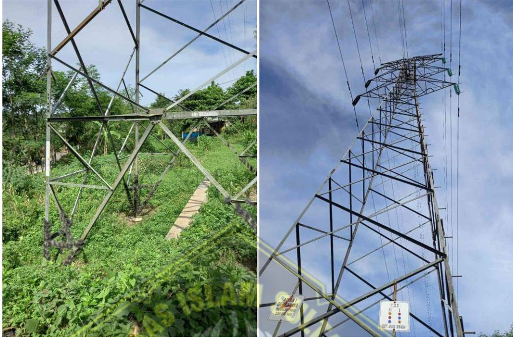
**Gambar 4.1. Kondisi Kaki Tower D23 SUTT 150kV Jelok-Bringin**
