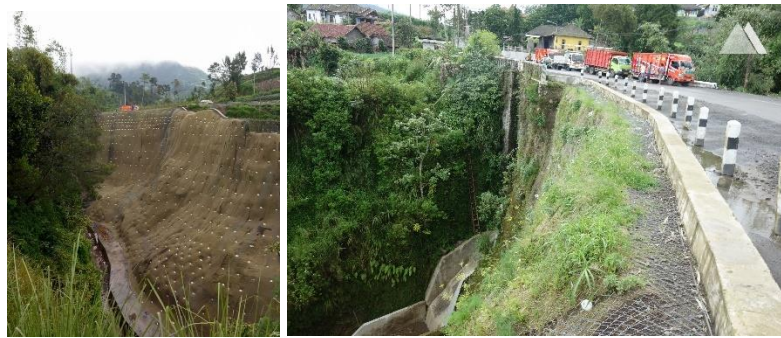
Gambar 2. 13 Soil Nailing di Jembatan Samiran 2 Boyolali Sumber: Selo Boyolali 2016 - Geobrugg, 2020
