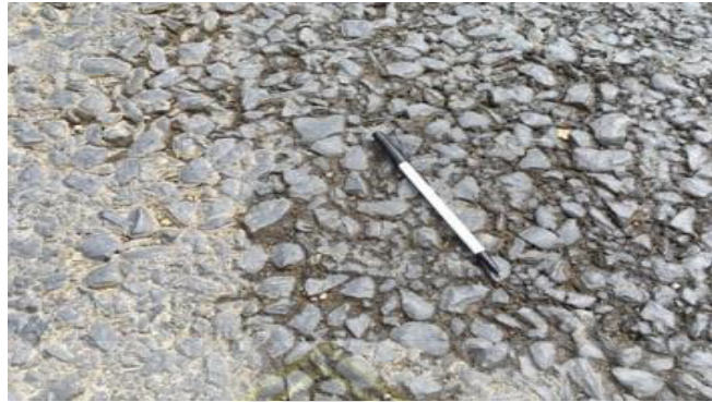
Gambar 2.19 Pengausan ( polished aggregate )
