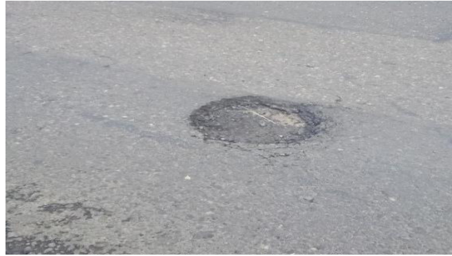
Gambar 2.16 Lubang ( potholes )
