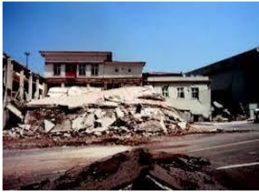
Gambar 2.8. Settlement Akibat Gempa Izmit, Turkey, 1999 (A.S. Elnashai, 2000)
