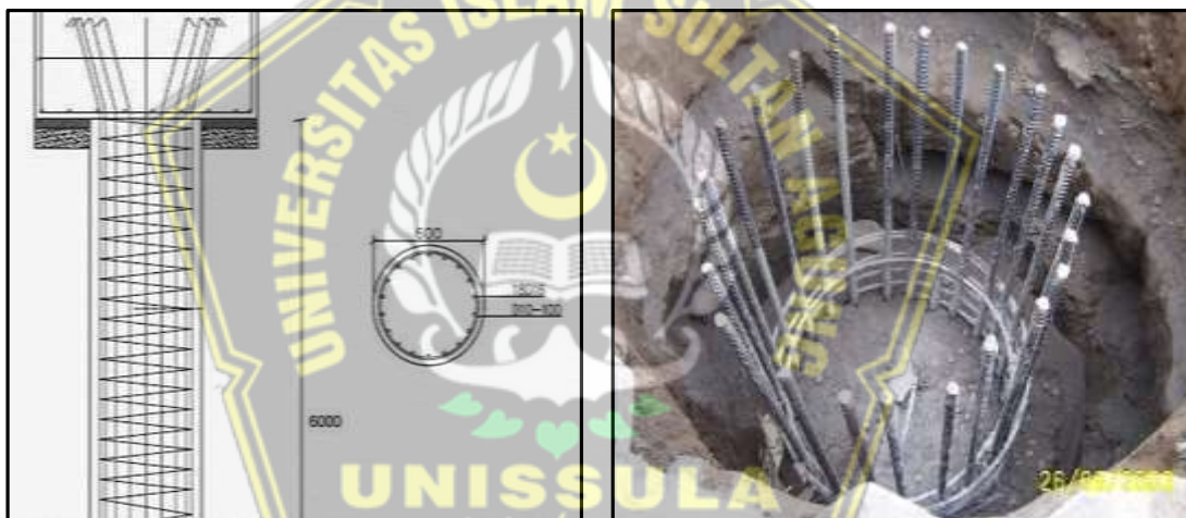
Gambar 2.1 Fondasi Bored Pile
