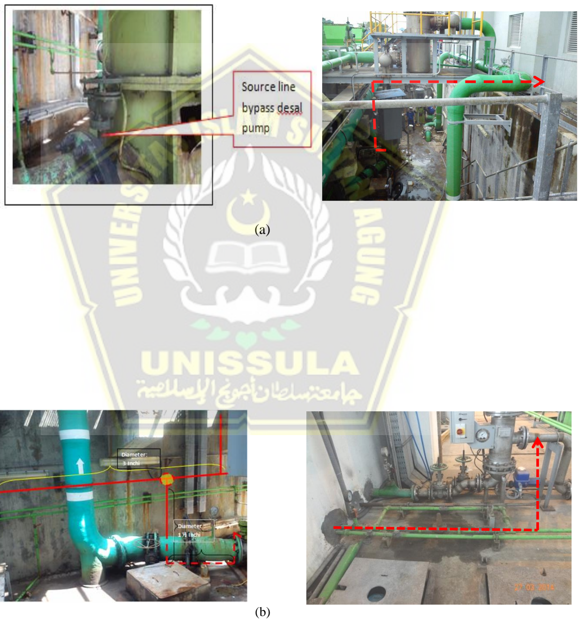
Gambar 4.6 Desain Jalur Pipa/Line Emergency Bearing Injection CWP
